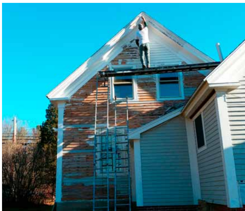
Torrey painting at work sealing up the Cowles house...
